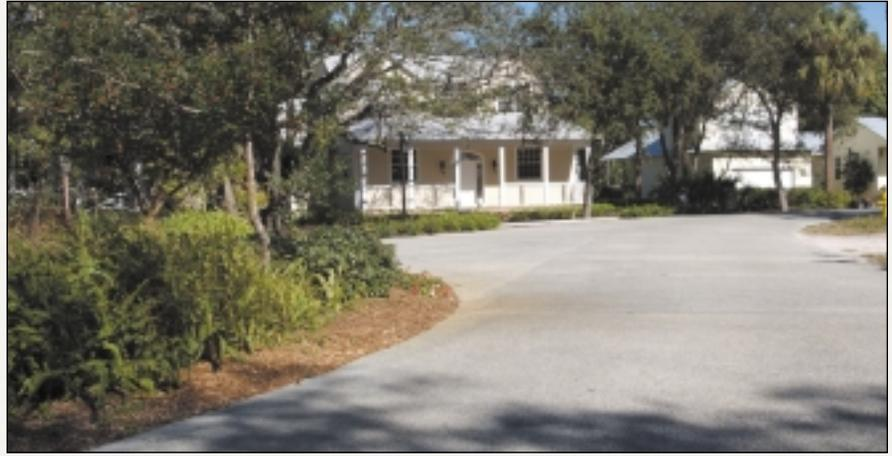
At Nature's Hideaway, the pervious pavement street was designed in center parts and running lanes. It is 20 feet across and 7 inches thick with 10 inches on the outside and a monolithic footer, angled down. The street paving was done all at one time, with the sidewalks and driveways added as homes were built.
